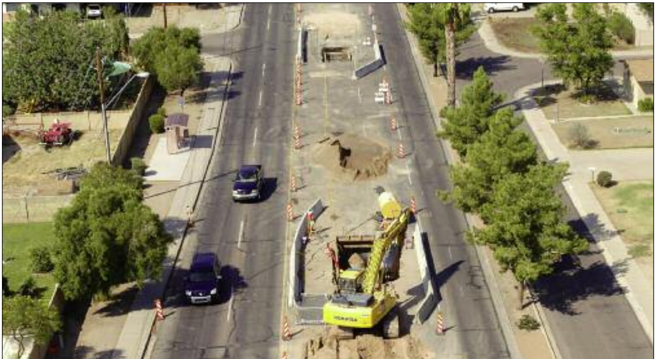
Peoria Avenue Pipe Burst- 375 mm (15 inch) to 450 mm (18 inch) VCP
