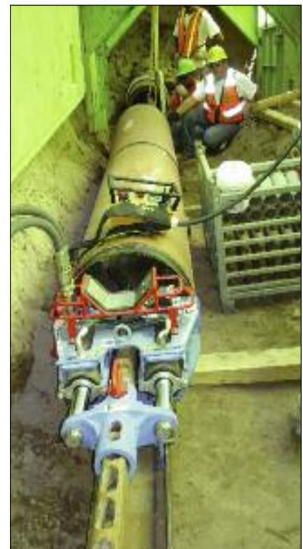
350 kN (40 ton) Cylinder Pack
